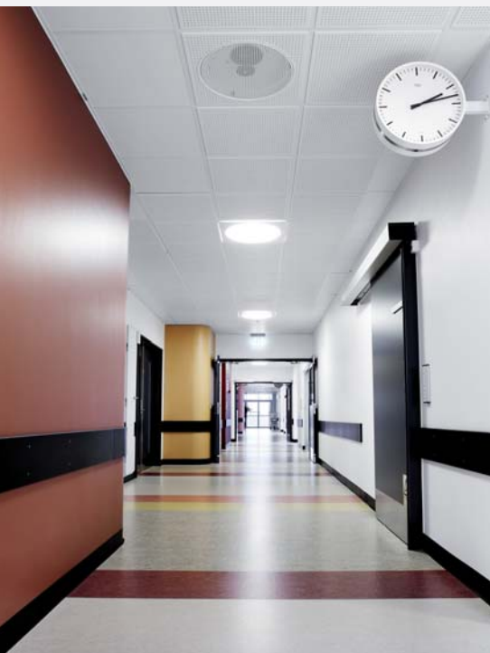
Korridor, Onkologisentret i Herning. Undertak: Gyptone Point 11 – kant E
